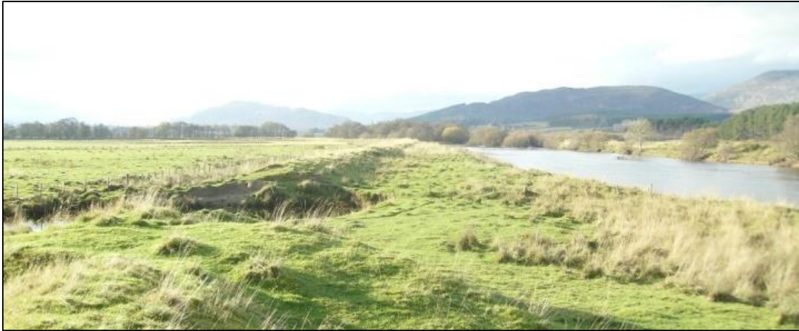
Figure C1: Breach scoured below level of adjacent channel bank.
